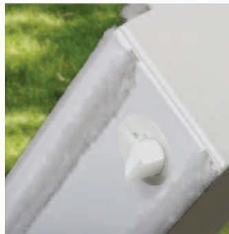
Tilt Latches (Vinyl Application)
